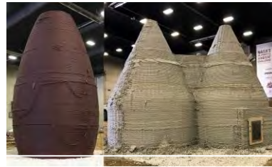
Fig. 2.2.2 - Left: MARSHA Right: Den@Mars, the two projects in the NASA 3D Printed Habitat Centennial Competition (Credit: IEEE Spectrum)
